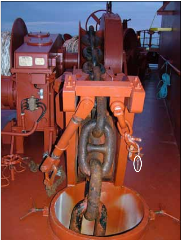
Senhouse slip securing pin in detached position
