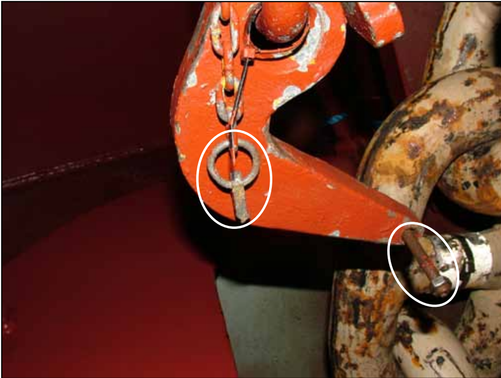
Maersk Newport's starboard anchor Senhouse slip failed tapered securing pin and replaced arrangement
