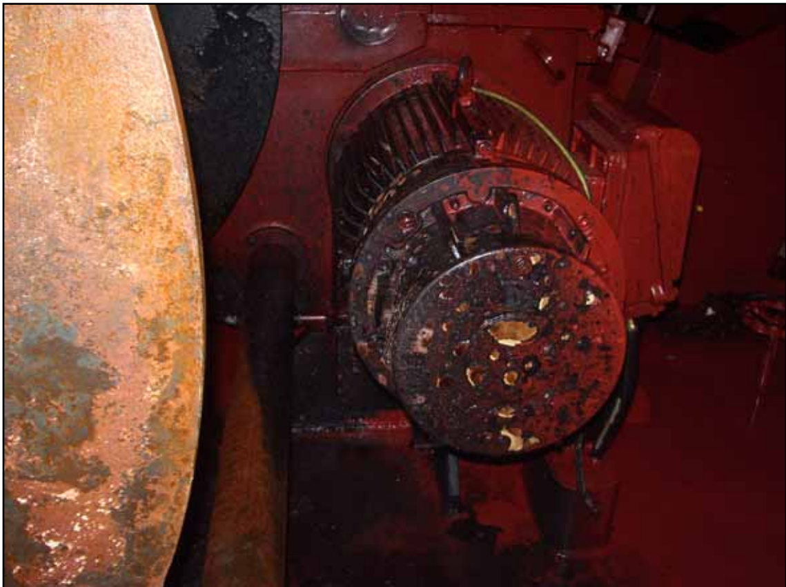
Fire damage to the port windlass winch
