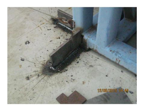
Welding of Lashing Stoppers on top of Hatch Covers
